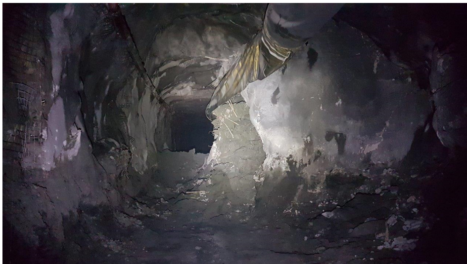
Figure 12 Large-scale plastic deformation in development at Diavik
