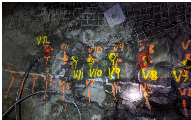
Figure 1 Example of the cable bolt trial area arrangement
