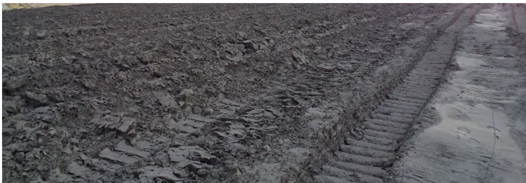
Figure 6 Filtered tailings material spread in layers 0.30 m thick
