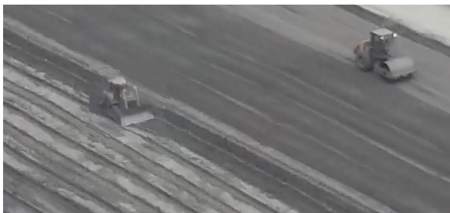
Figure 9 Compaction of filtered tailings
