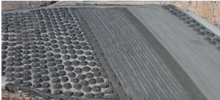
Figure 10 Compacted filtered tailings disposal cycle
