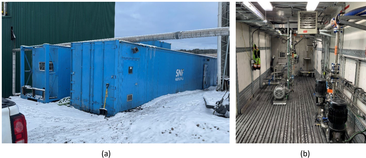
Figure 9 Various views of the unit at site. (a) Outside view; (b) Maturation tank and metering pump
