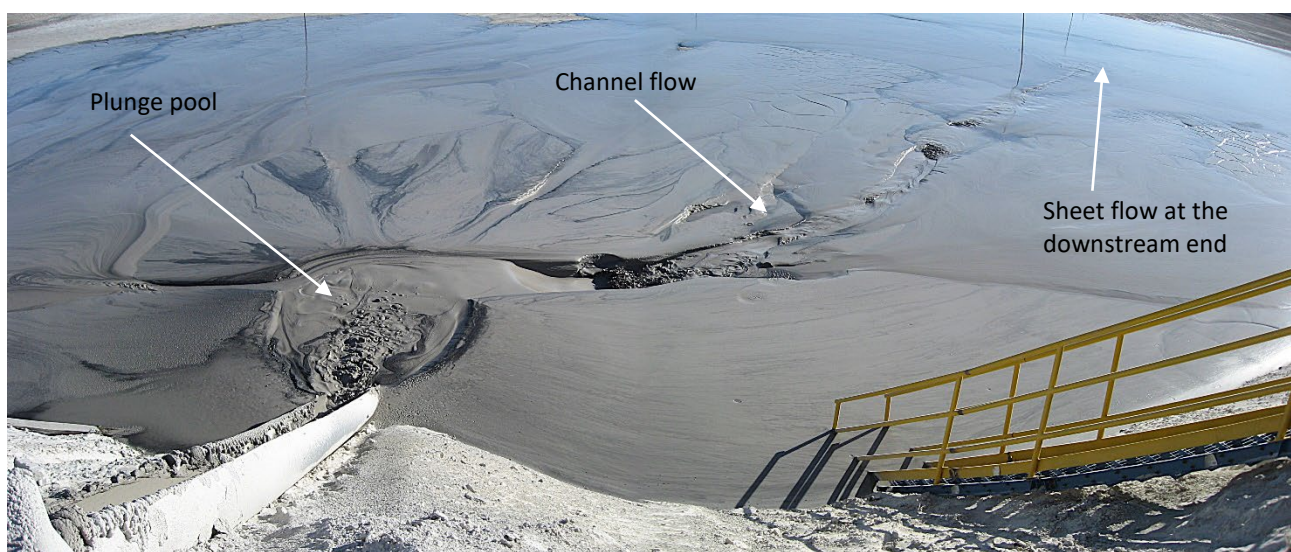
Figure 5 Stage 3 of beach formation. Establishment of the plunge pool and channelised flow in the preferred direction
