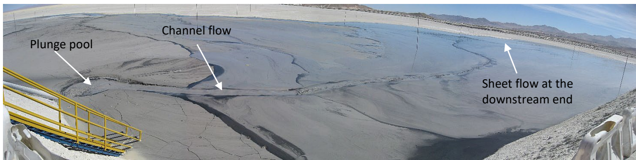
Figure 6 Stage 4 of beach formation. Further advancement of the tailings beach toward the downstream area
