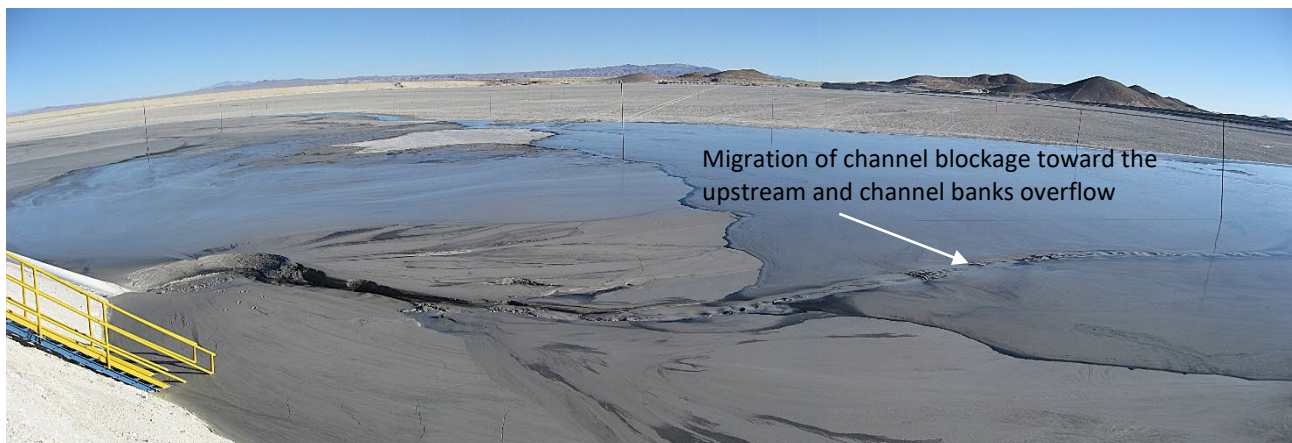
Figure 7 Stage 5 of beach formation. Gradual blockage of the channel flow from the downstream deposition
