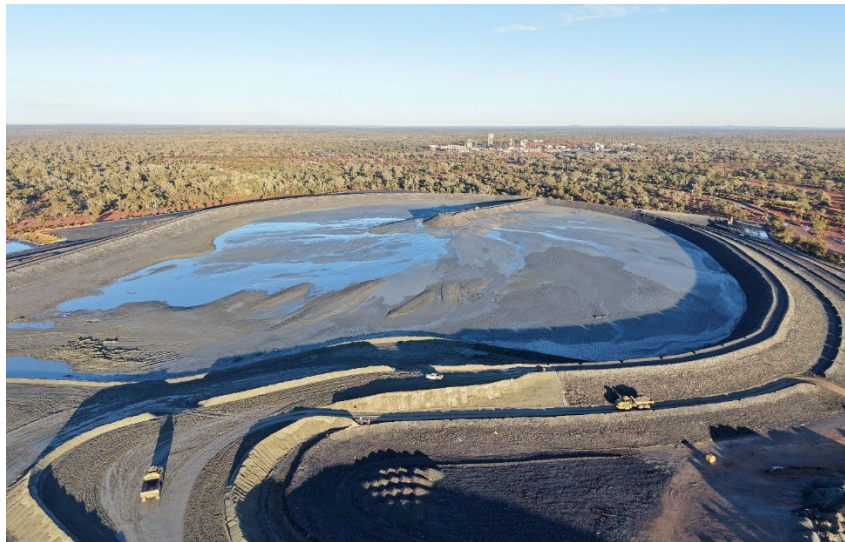
Figure 1 Tailings deposition onto west mound following Stage 10 raise construction
