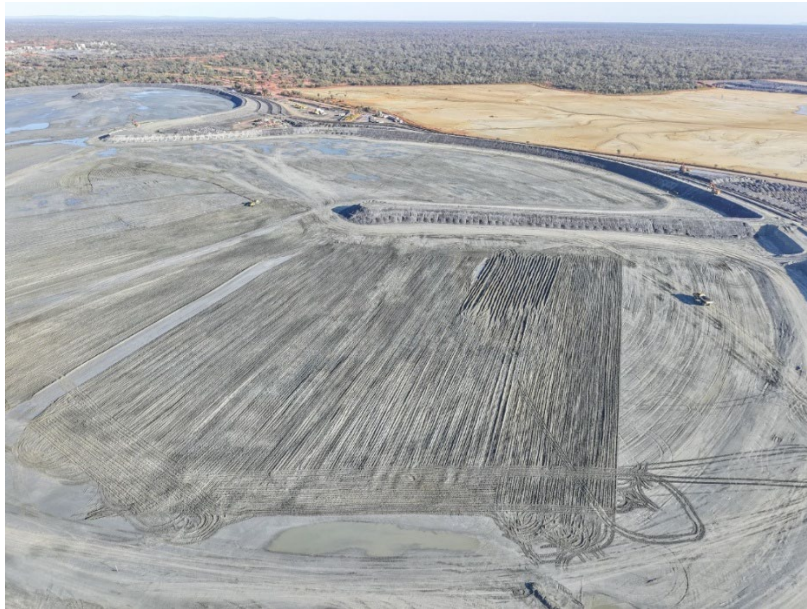
Figure 6 Shaped east mound tailings borrow pit
