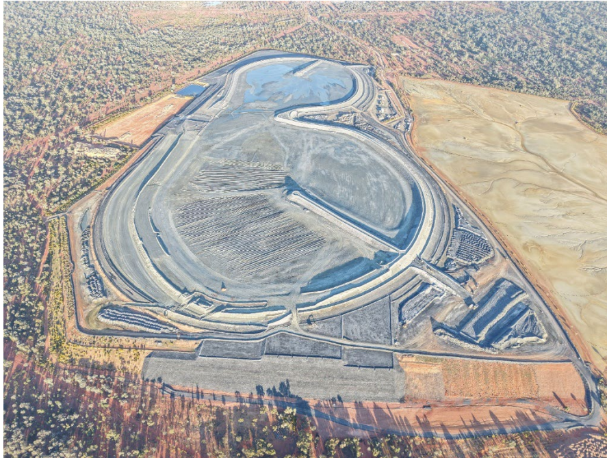
Figure 4 Westward view across the east and west tailings mounds during Stage 10 raise construction
