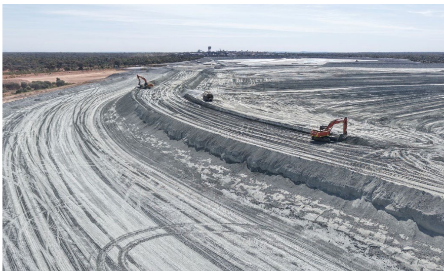
Figure 5 Stage 10 top-hat raise construction over widened embankment adjacent to decant area
