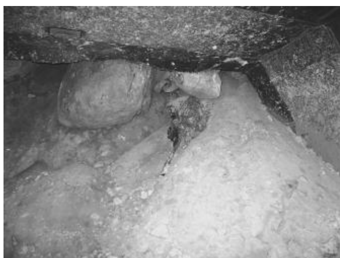
Figure 6 Mesh and bolt in P9-11W
