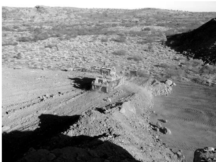
Figure 11 D10 bulldozer pushing lower slope of constructed mesa landform
