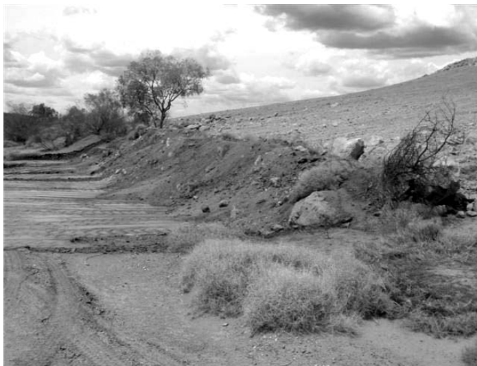
Figure 15 Repairs to shoulder of Rudall River Road
