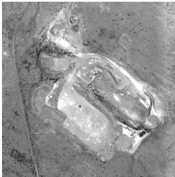
Figure 5 Aerial view of Pit 13 (pre-rehabilitation)
