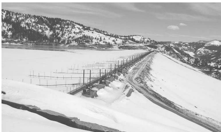
Figure 1 Cyclone sand dam construction
