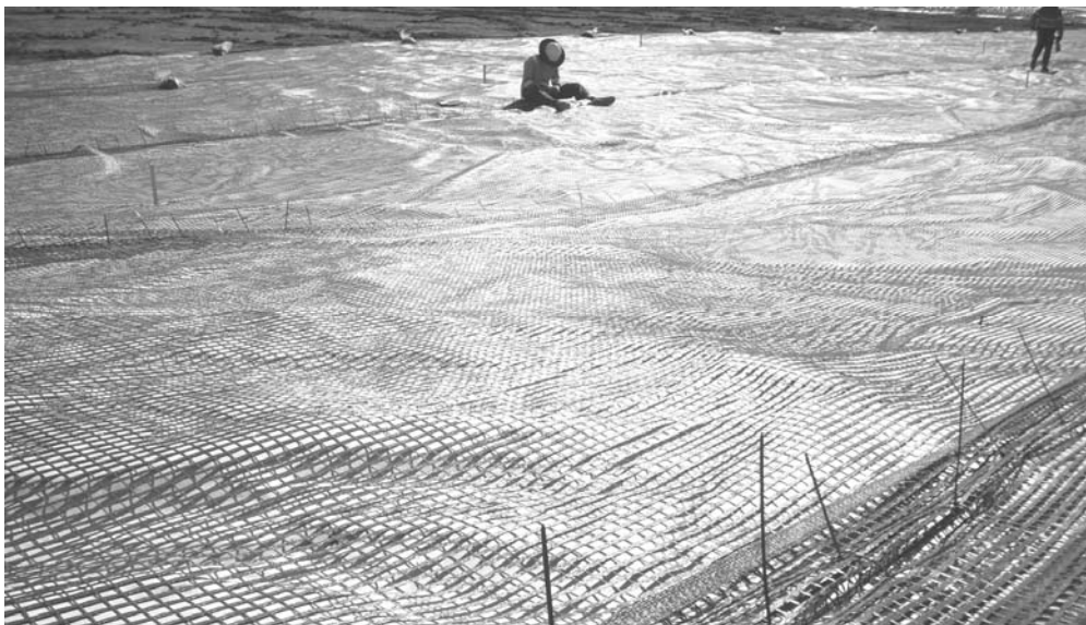
Figure 16 Photograph of stitching of geogrid seams with cable ties
