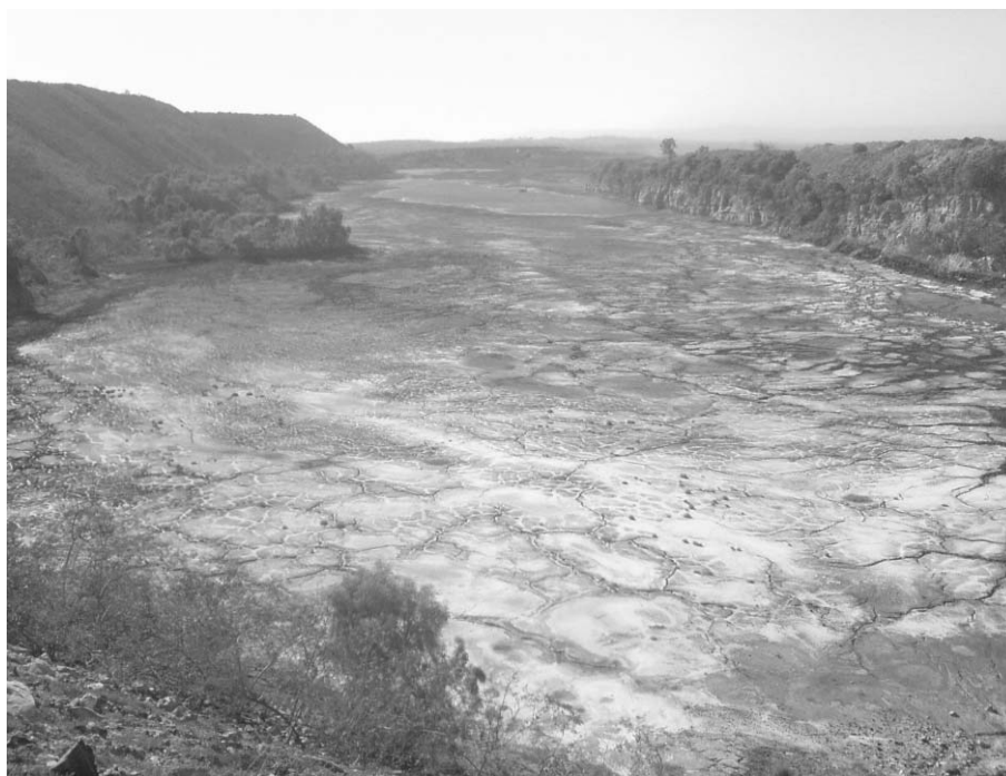
Figure 1 Wambo NE TD prior to commencement of capping operations
