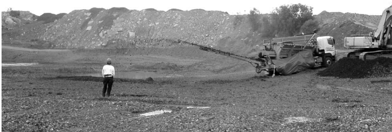
Figure 17 Photograph of slinger conveyor truck placing infill between fingers
