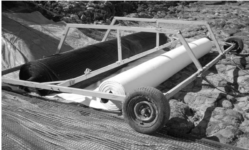
Figure 15 Photograph of dolly for placement of geosynthetic material
