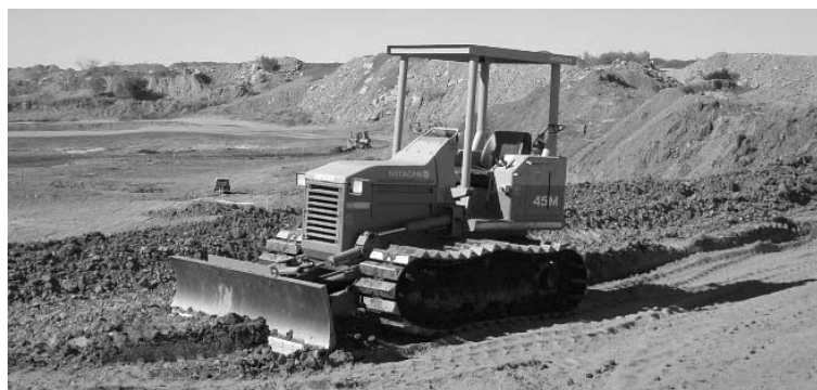
Figure 13 Photograph of a dozer equivalent to a D2, with low ground pressure tracks. This machine has been used to push mixed reject material onto the NE TD in fingers
