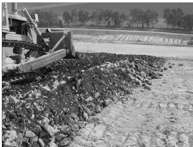
Figure 8 Placing rock-mulch cover
