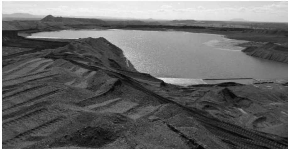
Figure 3 Pumped co-disposal – coarse rejects containment with tailings contained in the middle
