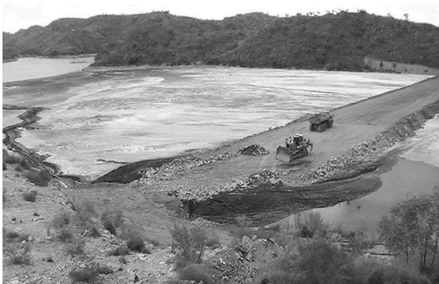
Figure 17 Groyne No. 9 near completion to full height
