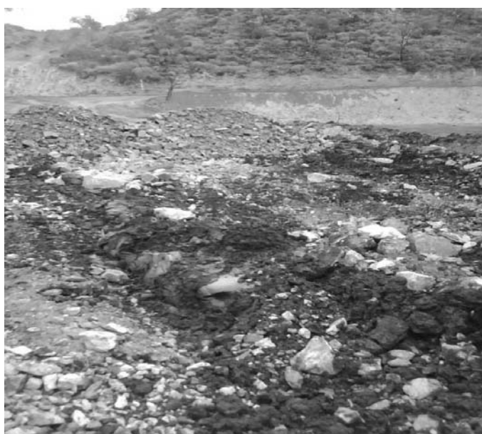
Figure 13 Typical penetration of tailings – push into tails
