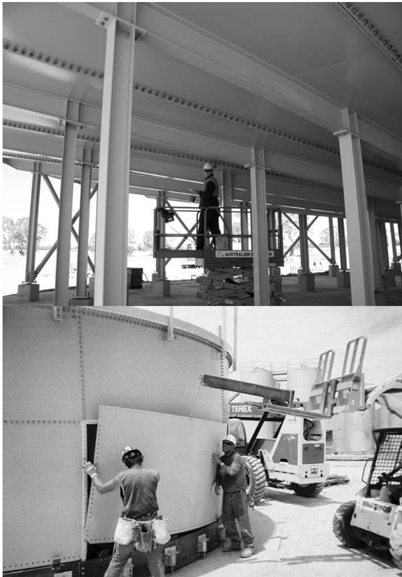
Figure 2 Flanged joints on thickener (top) versus lap joints on water tank (bottom)
