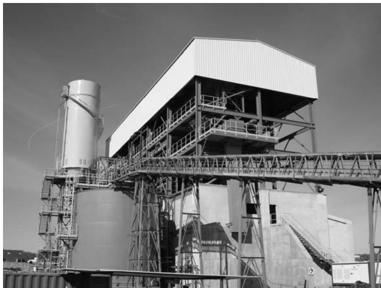
Figure 1 Aguas Tenidas paste backfill plant, Spain
