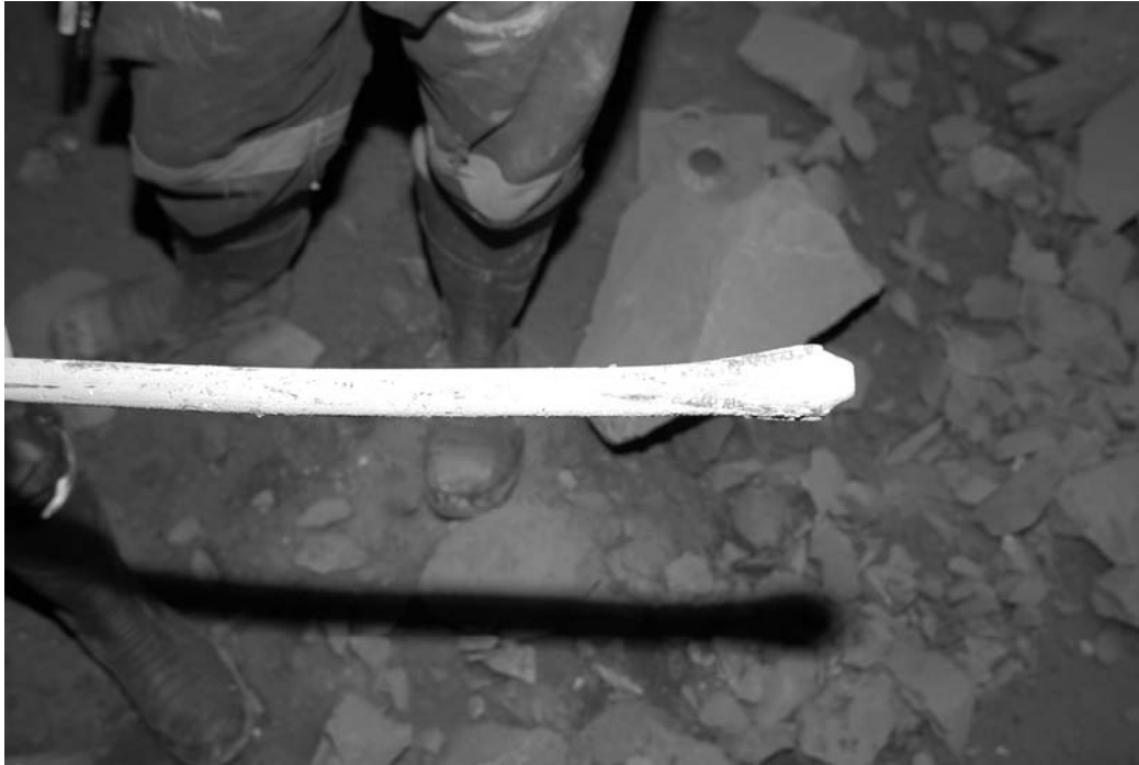
Figure 15 Cone bolts pulled out of the grout during the second blast
