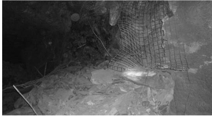
Figure 5 Damage of pillar nose on 5100 Level
