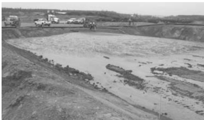
Figure 5 Early deposition in a cell, looking towards central staging area
