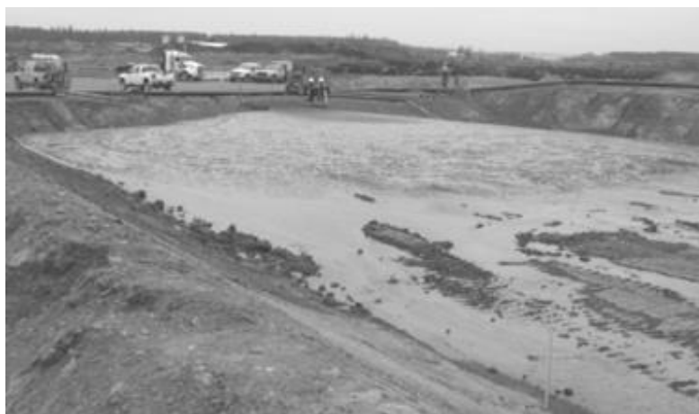
Figure 5 Early deposition in a cell, looking towards central staging area
