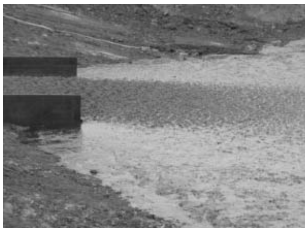
Figure 4 Amended MFT pouring out of spill box
