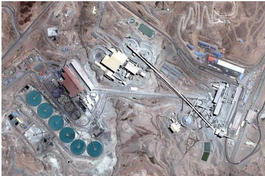
Figure 1 General view of the productive system (source: Google Earth)
