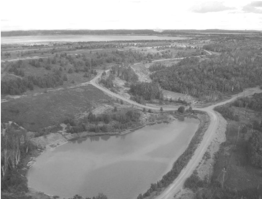
Figure 3 Photo showing vegetation on an Old Stack tailings beach and dam slope and a seepage pond with P Area Pond in the background
