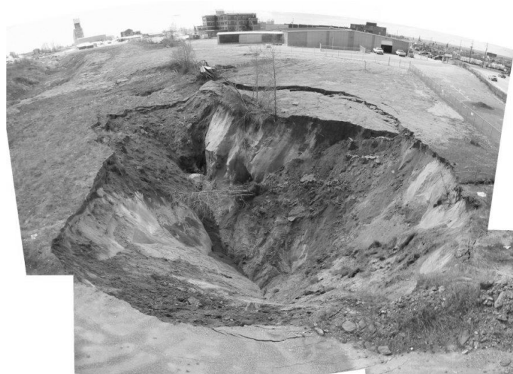
Figure 2 Subsidence near downtown Timmins
