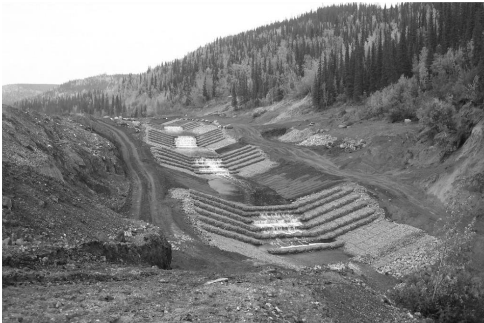
Figure 5 Completed channel stabilisation works (2004)
