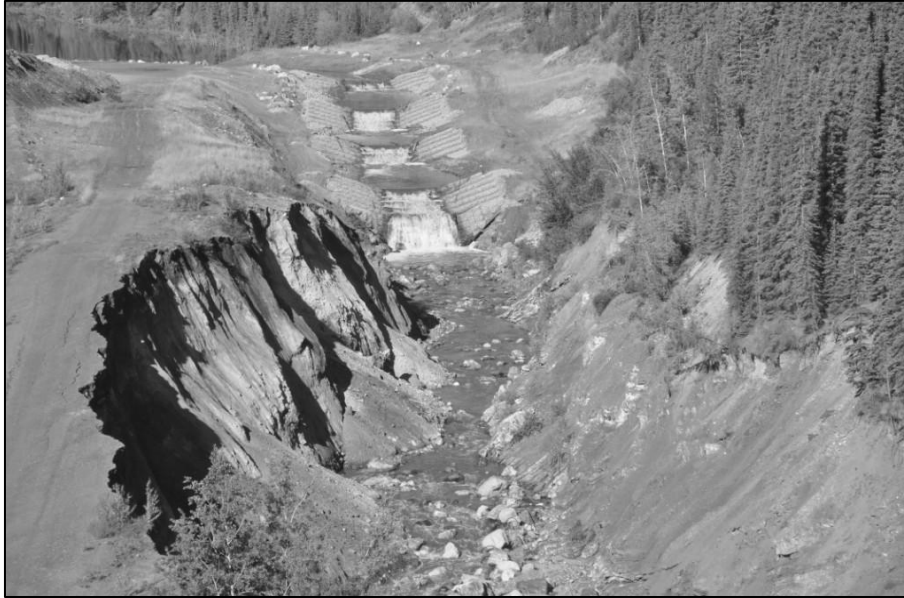
Figure 6 Clinton Creek Channel d/s of DS#4 on August 23, 2010
