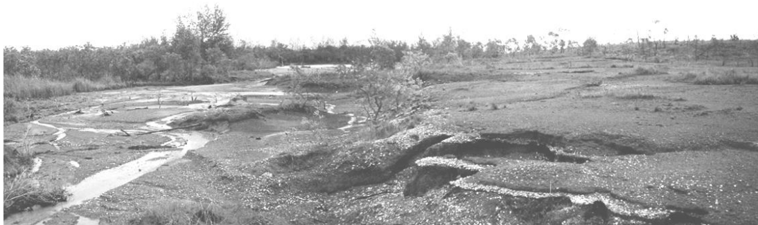
Figure 2 Southern edge of Taylor's Pond at Rio-Tinto Alcan Gove's red mud pond system. Note the underscoring of the poorly vegetated and stabilised surface
