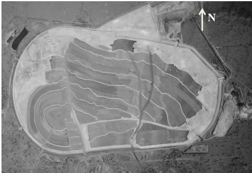
Figure 2 Aerial photo of Pillara TSF showing rock barrier contours
