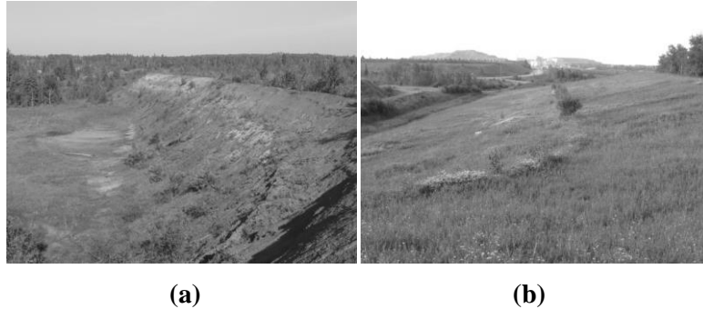
Figure 3 Tailings dam slope re-grading: (a) prior to re-grading; (b) after re-grading
