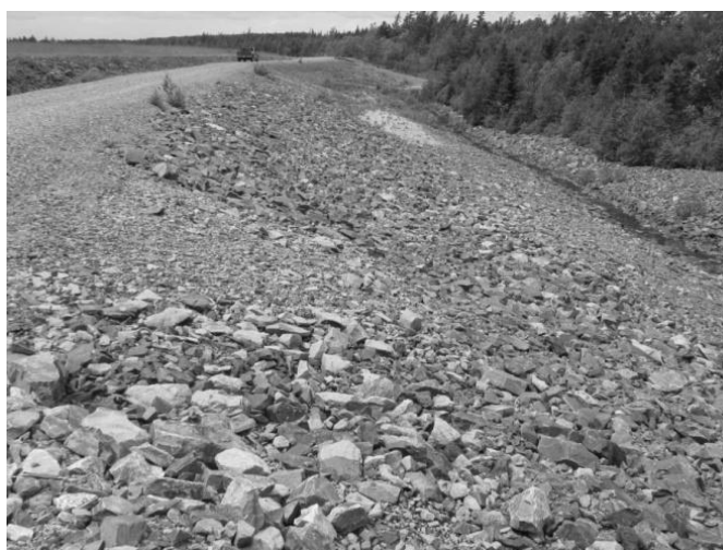
Figure 6 Rockfill is typically used as erosion protection on dam surfaces
