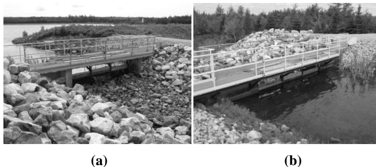
Figure 9 Typical stoplog structure: (a) downstream view; (b) upstream view
