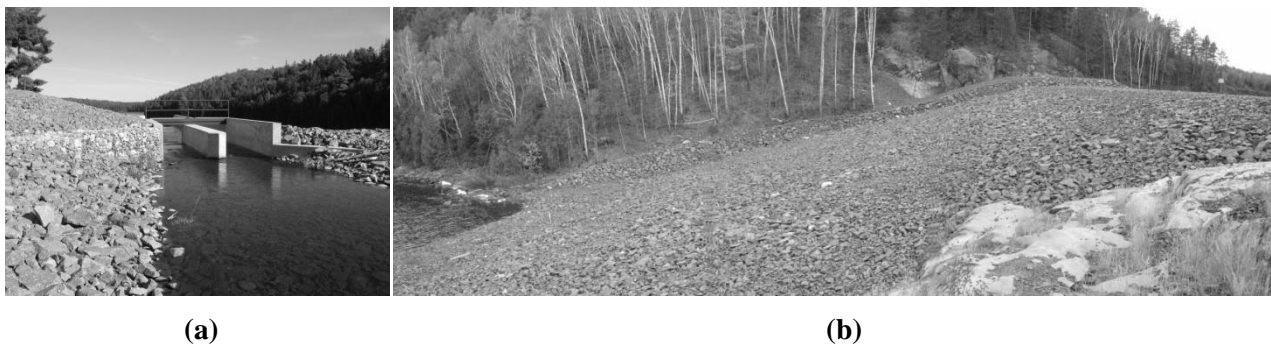
Figure 11 (a) Decant channel; (b) storm spillway
