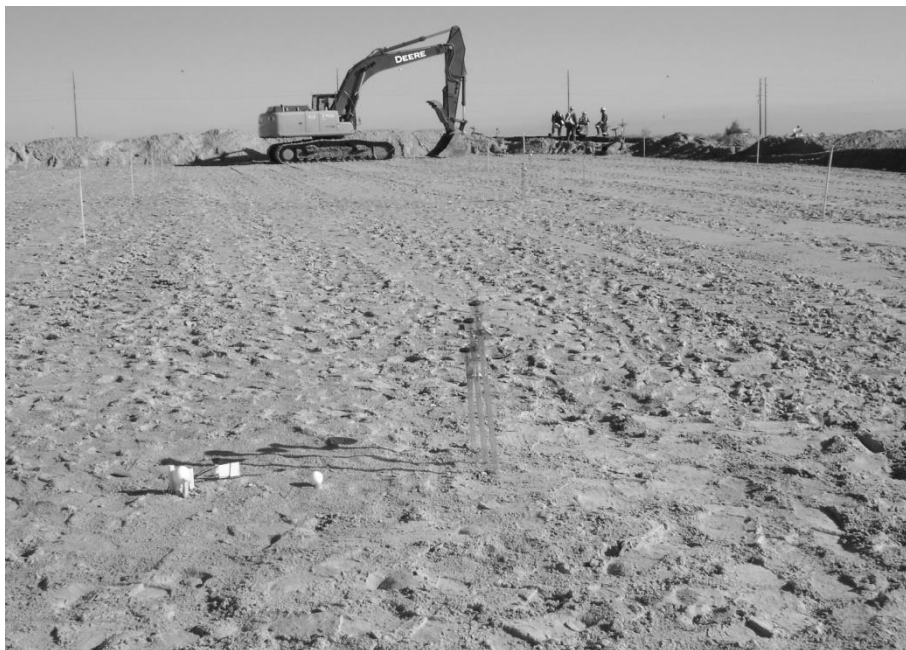
Figure 1 Construction and instrumentation of a sand bermed cell (50 m x 100 m)
