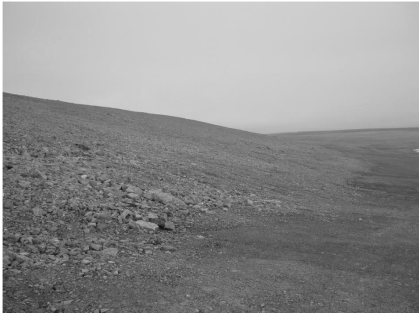
Figure 4 Rock fill cover, operational landfill, former Polaris Mine, Nunavut (photo courtesy D. Johnson (with permission of Teck Resources Ltd.))
