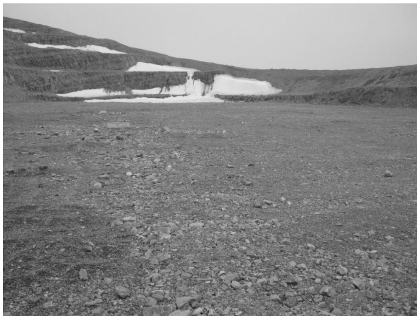
Figure 3 Rock fill cover, Little Red Dog Quarry landfill, former Polaris Mine, Nunavut (photo courtesy D. Johnson (with permission of Teck Resources Ltd.))
