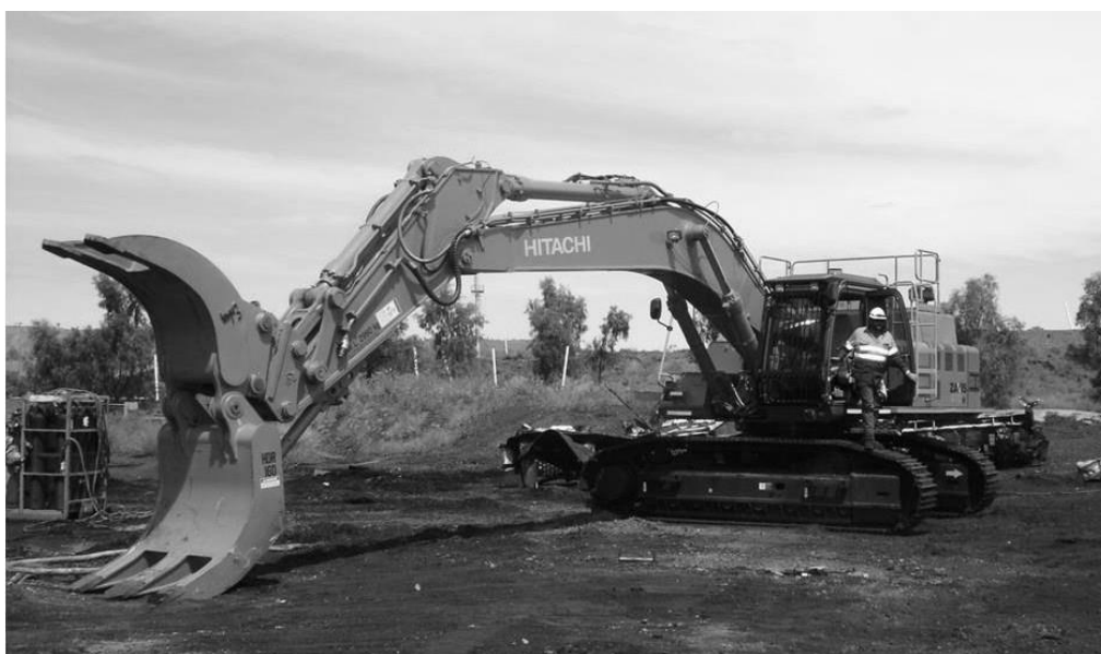
Figure 3 A 47 tonne excavator with grab attachment
