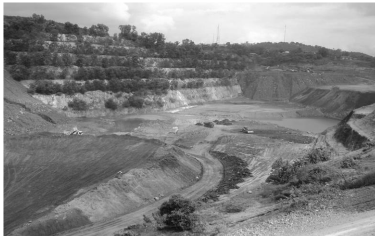
Figure 13 Backfilling the GSBPL plant north pit
