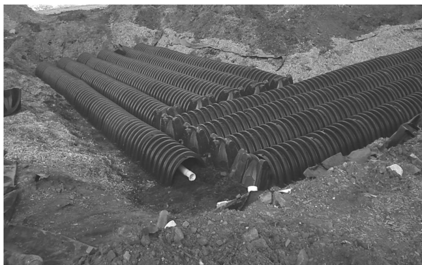
Figure 4 Influent dispersion chambers during retrofit
