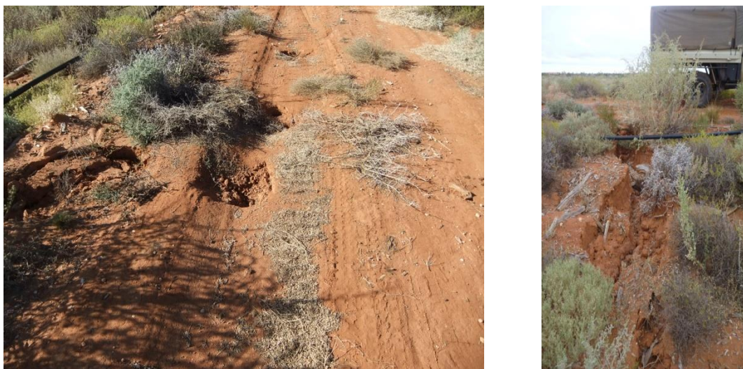
Figure 11 Runoff discharging from perimeter track onto outer batter and causing scour
