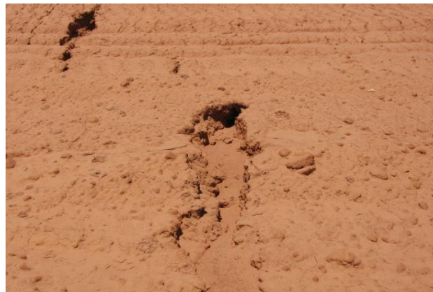
Figure 3 Tunnel erosion on waste dump batter
