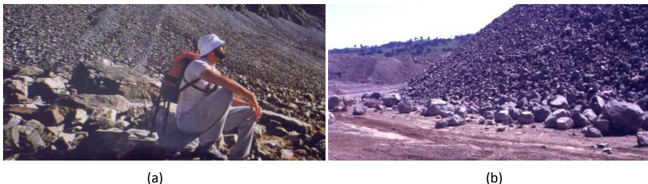
Figure 5 Formation of base rubble zone of a surface waste rock dump: (a) Natural rock slope, and (b) Waste rock dump slope
