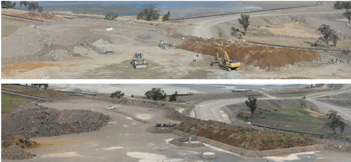
Figure 10 Views of top of Cadia trial waste rock dump; top: at the completion of construction in February 2006; bottom: 18 months later in August 2008
