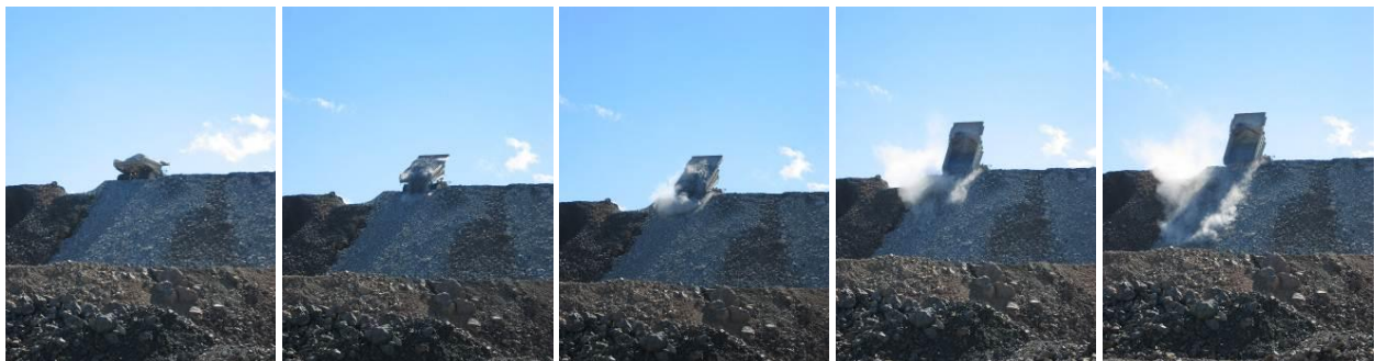
Figure 3 Sequence of end-dumping off a surface waste rock dump tip-head
