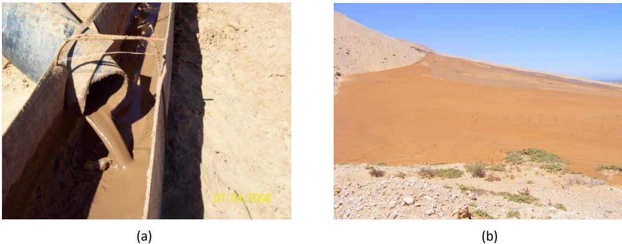
Figure 4 (a) Launder systems for underflow transportation; (b) slope flattening in progress
