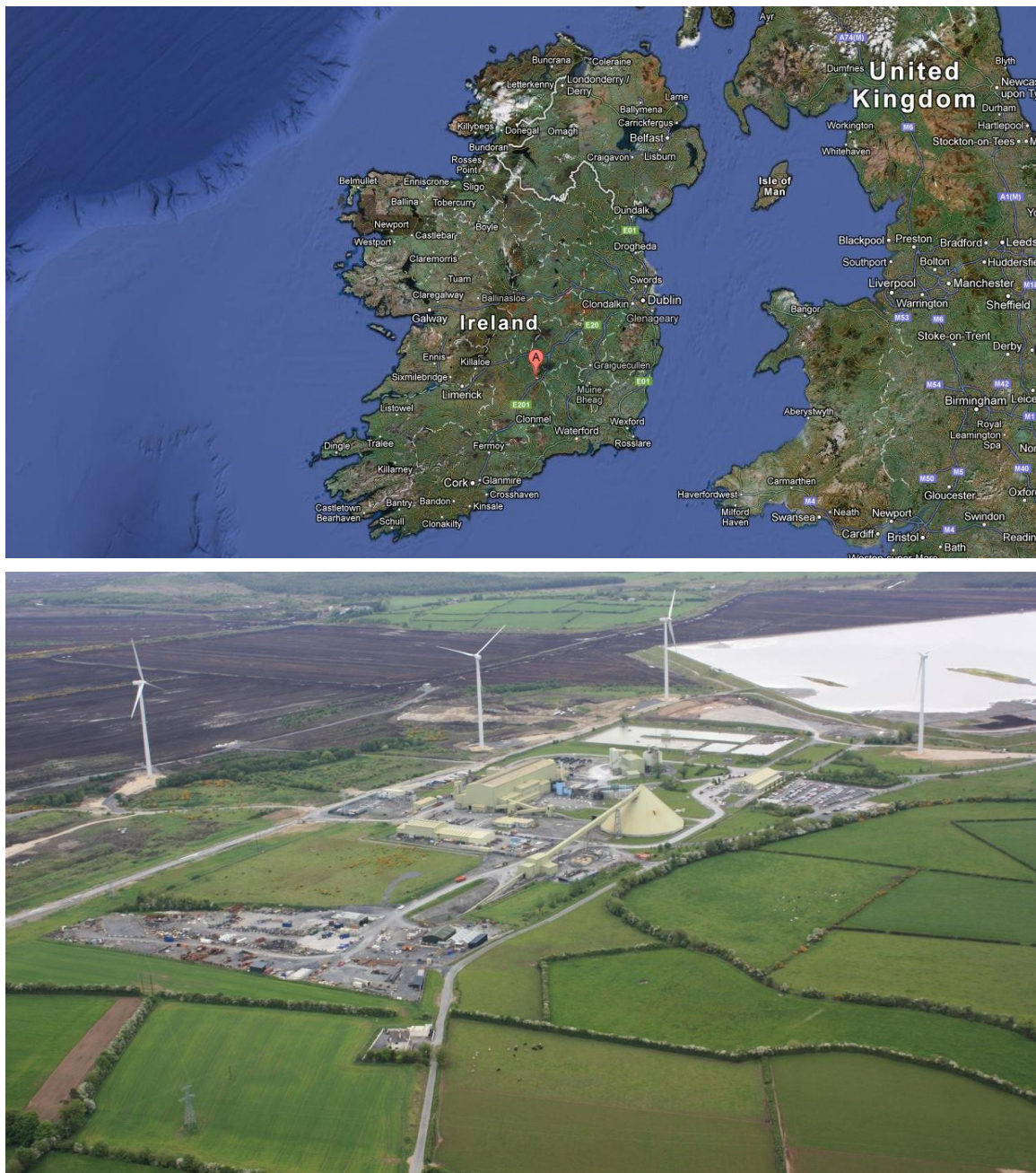
Figure 1 Lisheen Mine, Co. Tipperary, Ireland location and aerial photograph
