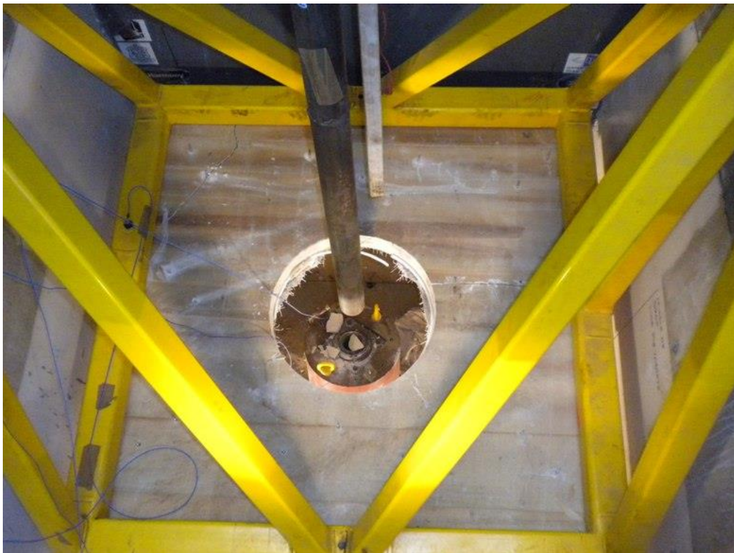
Figure 11 Punch through failure for sample 4
