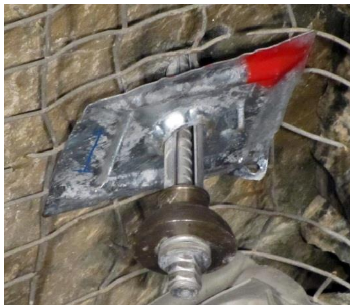
Figure 5 A bolt collar after being tested
