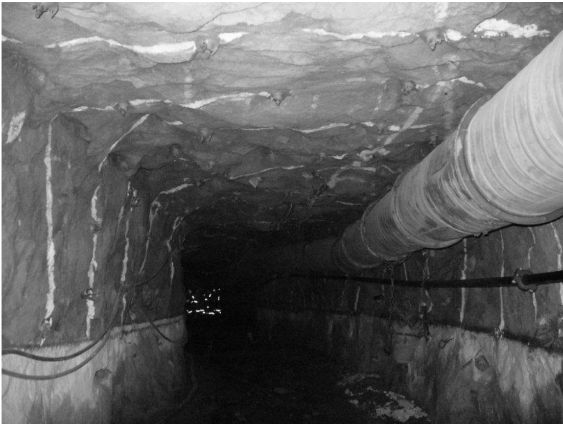
Figure 4 Typical Bushveld ground conditions and support pattern (photo not from Impala)
