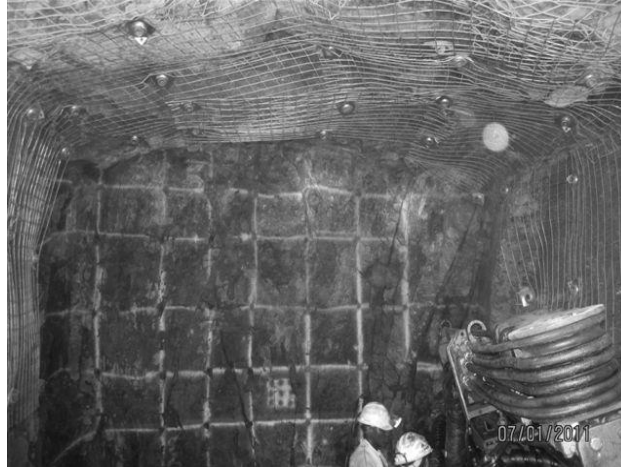
Figure 9 Showing welded mesh and friction stabilisers installed in shallow blocky ground conditions
