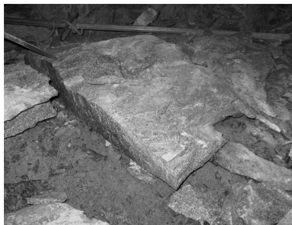
Figure 7 Thick 'slab' type stress-fractured block in noritic rock type at No. 17 shaft
