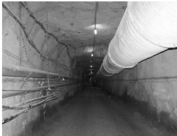
Figure 10 Showing fibrecrete and resin-grouted rebars in deep, fractured ground conditions
