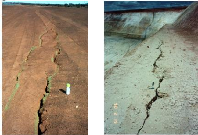
Figure 6 Extension cracks; (left) in the ground surface behind the crest of an open pit wall; (right) in a bench within a pit wall (photographs M.C. Bridges)
