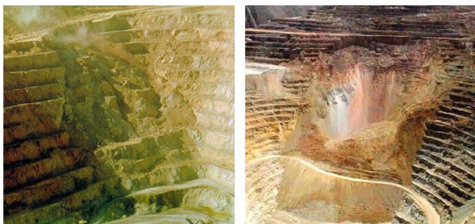
Figure 9 Large-scale failures in walls of open pits; (left) structural control by faults is evident at the top, but the mechanism in the lower part is unclear; (right) evidence of faults at the back of the failure, but the trigger of the failure was unclear (Hoek et al., 2000)
