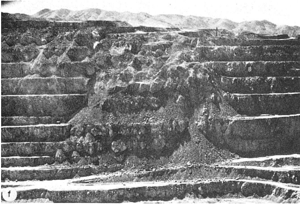
Figure 4 View of the Chuquicamata pit wall after the initial clean-up of the collapsed rock (from Voight and Kennedy, 1979)
