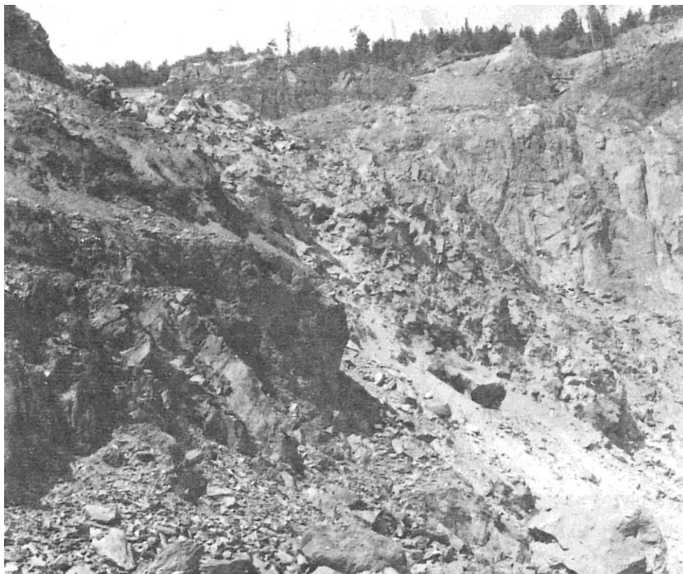
Figure 2 Instability and failure of a pit wall that was claimed to have failed by initiation by shearing at the toe followed by a breakdown of the rock mass (Coates and Yu, 1978)
