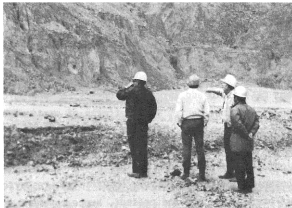
Figure 7 Heave of the floor of about 1 m near the toe of a 90 m high pit wall (from Coates and Yu, 1978)
