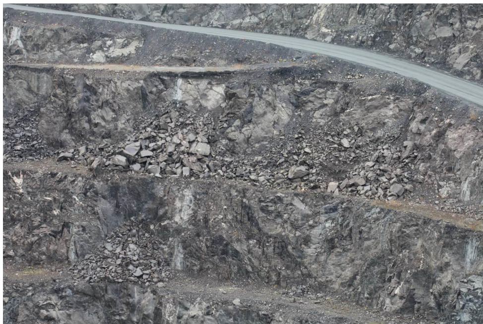
Figure 5 Wedge type failures in northwest – part of the main pit
