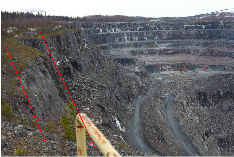
Figure 6 Planar type failure in east pit wall. Most of the shear zone has collapsed
