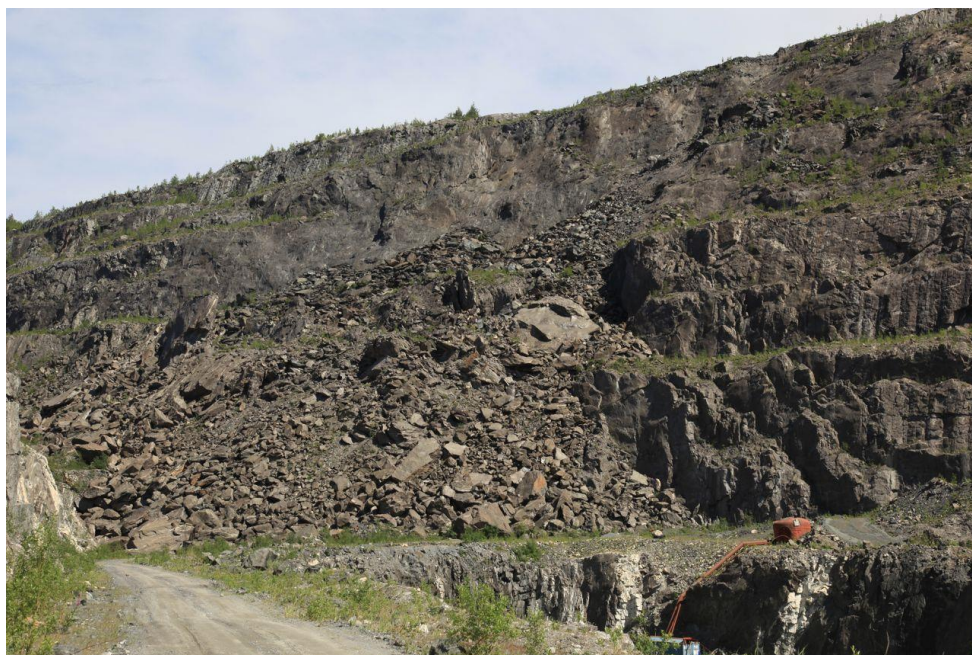
Figure 7 Pit wall failure (April 2002) in northeast – part of the main open pit caused by the major shear zone in the east wall
