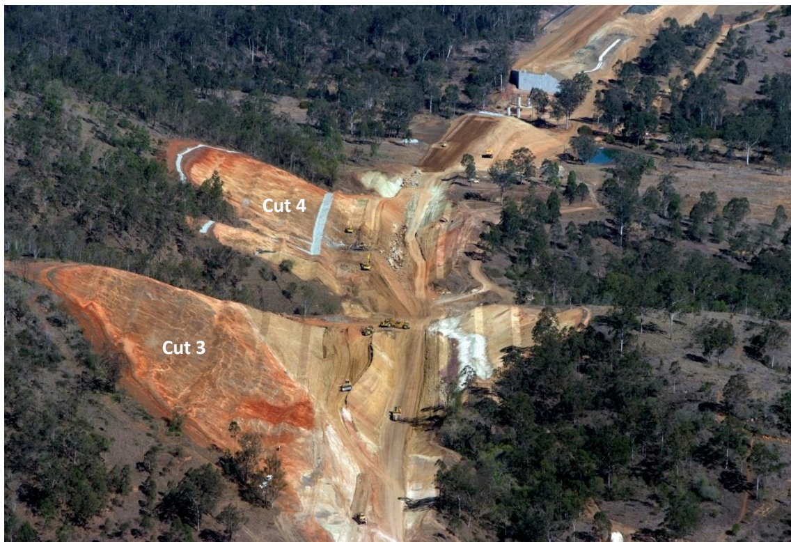
Figure 1 Aerial view of Cut 3 and Cut 4 during construction (2007)
