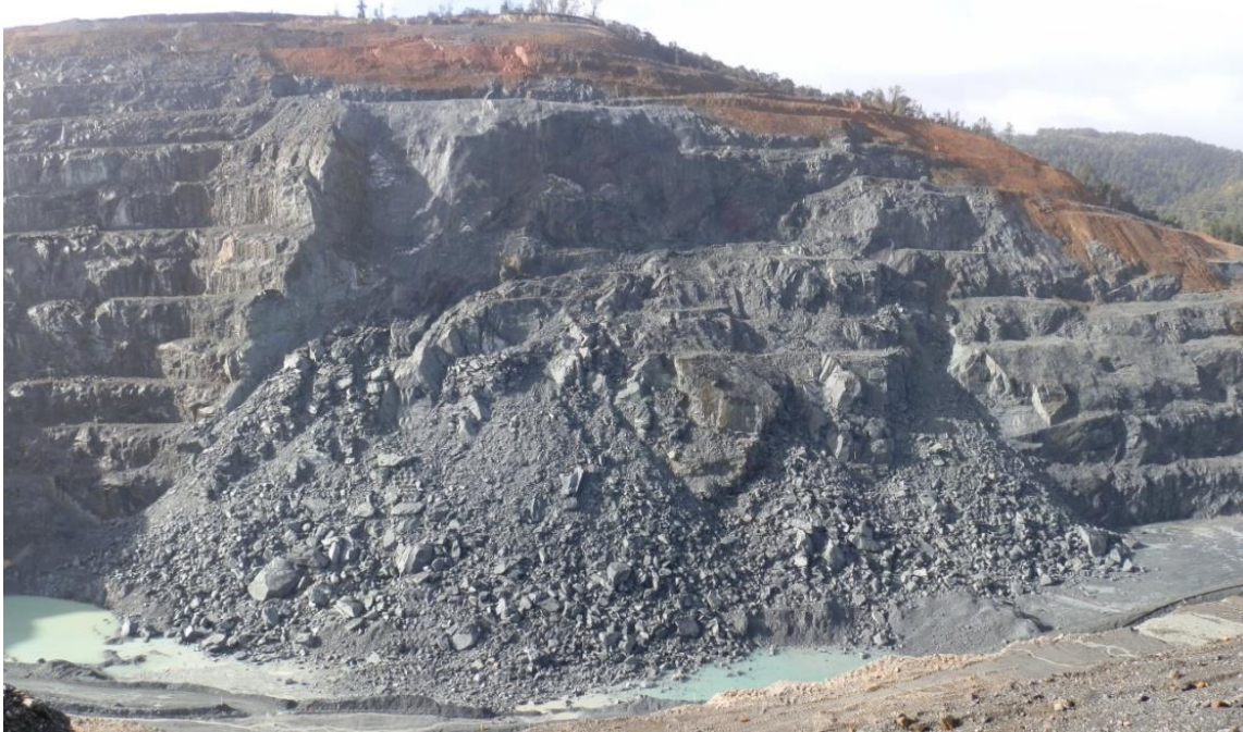
Figure 6 July 2012 east wall failure
