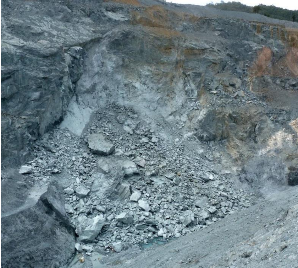
Figure 7 November 2012 east wall failure
