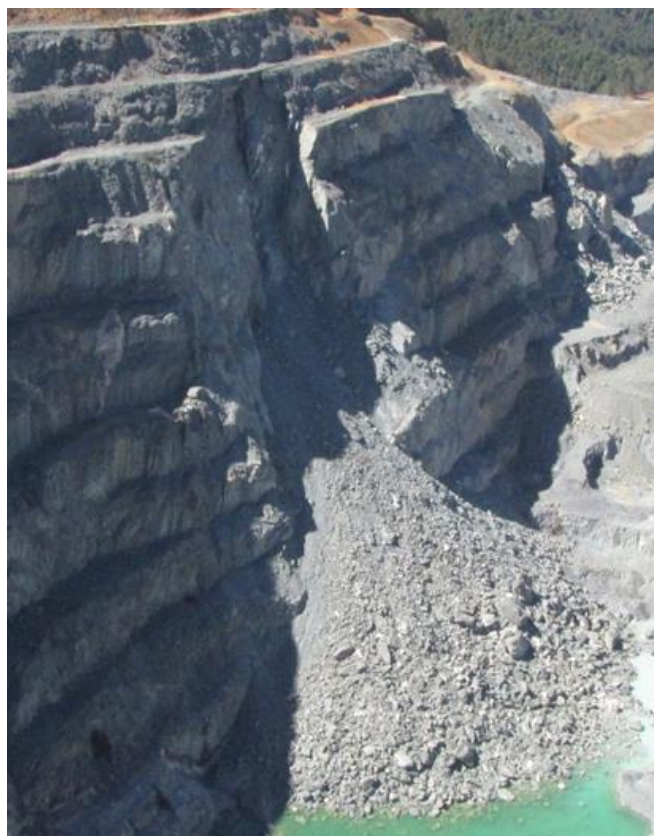
Figure 4 June 2010 east wall failure
