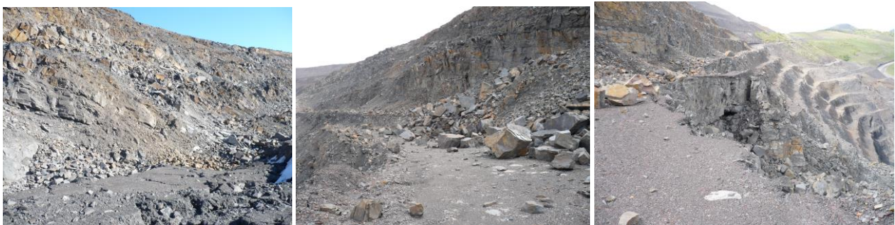
Figure 4 Degradation in an area of the eastern slope
