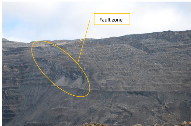
Figure 5 Eastern slope fault area
