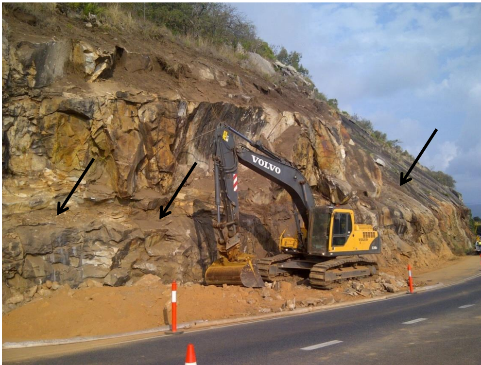
Figure 2 View of the northern section of the Rex Lookout site. The exfoliation joint exposed in the cutting extends to form the natural ground surface to the rear of the excavator
