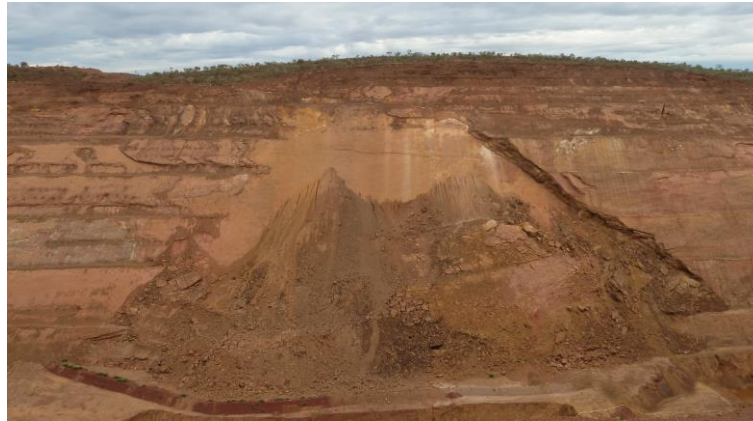
Figure 12 CEPN 2010 slope instability
