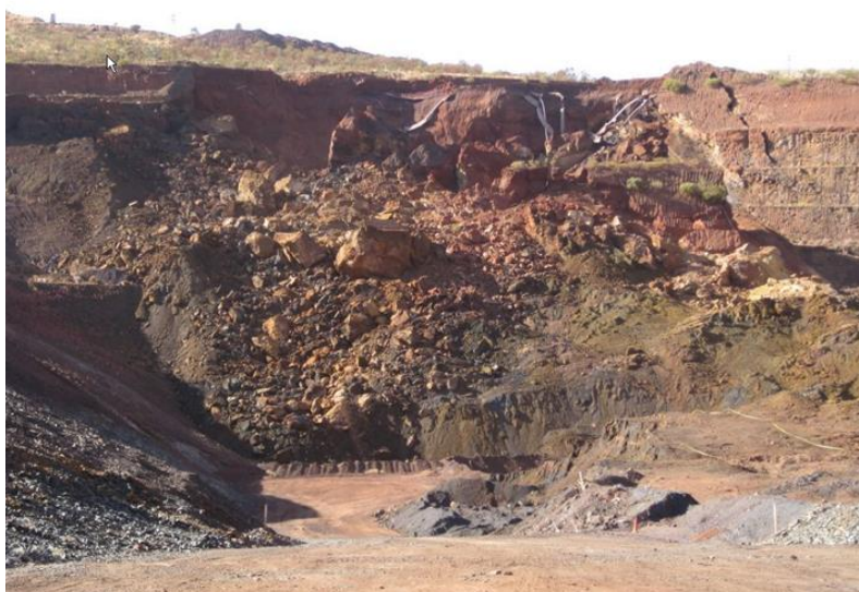
Figure 1 NTD 2009 slope instability
