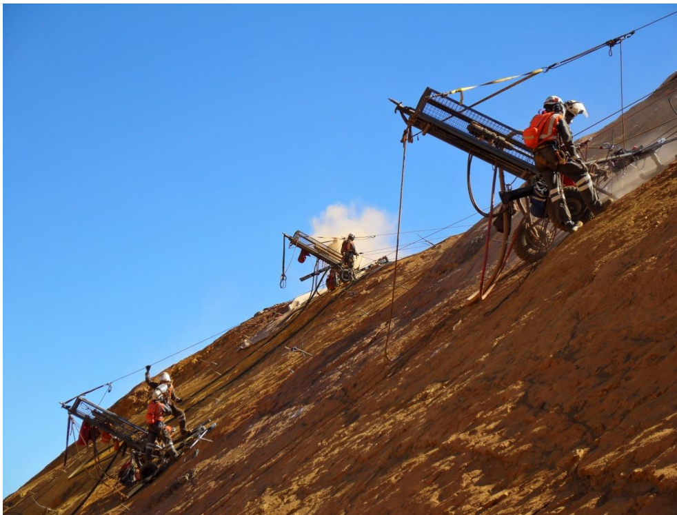
Figure 8 Rope-access drilling with light weight drill rigs at 150 m above the pit base
