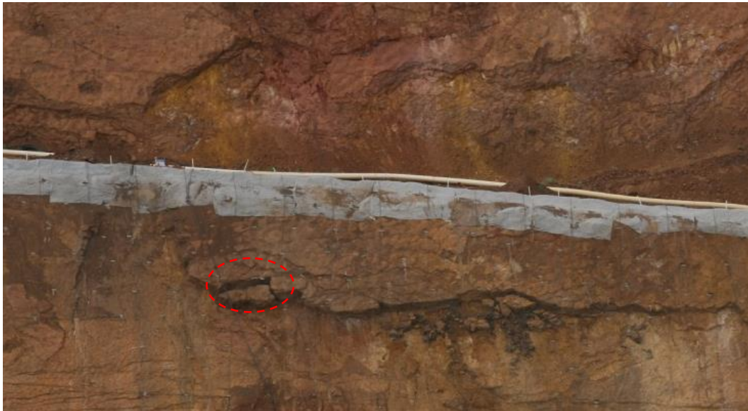
Figure 9 Location of loosened boulders retained by the TECCO mesh system
