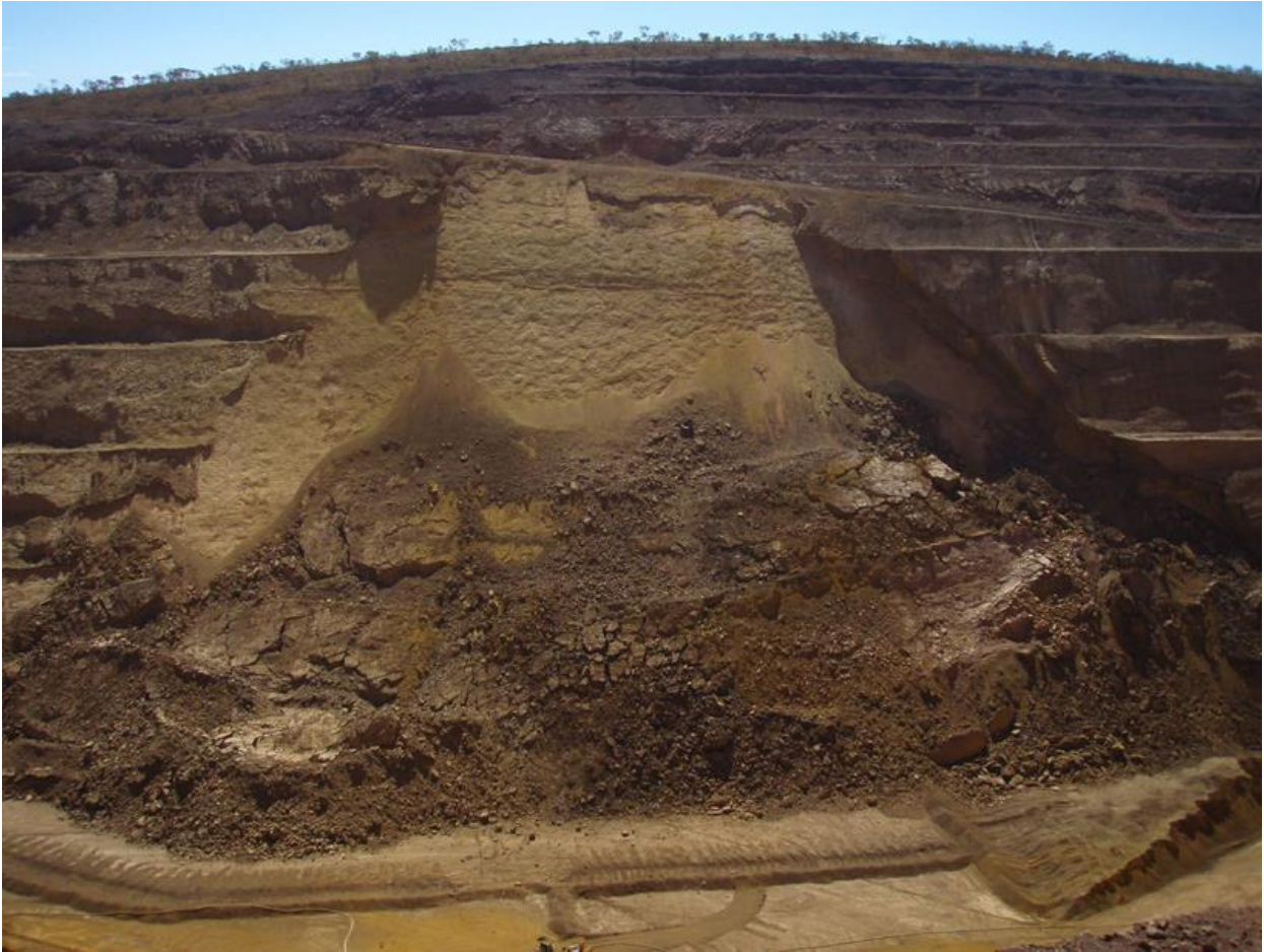
Figure 1 Major slip failure at north wall, West Angelas
