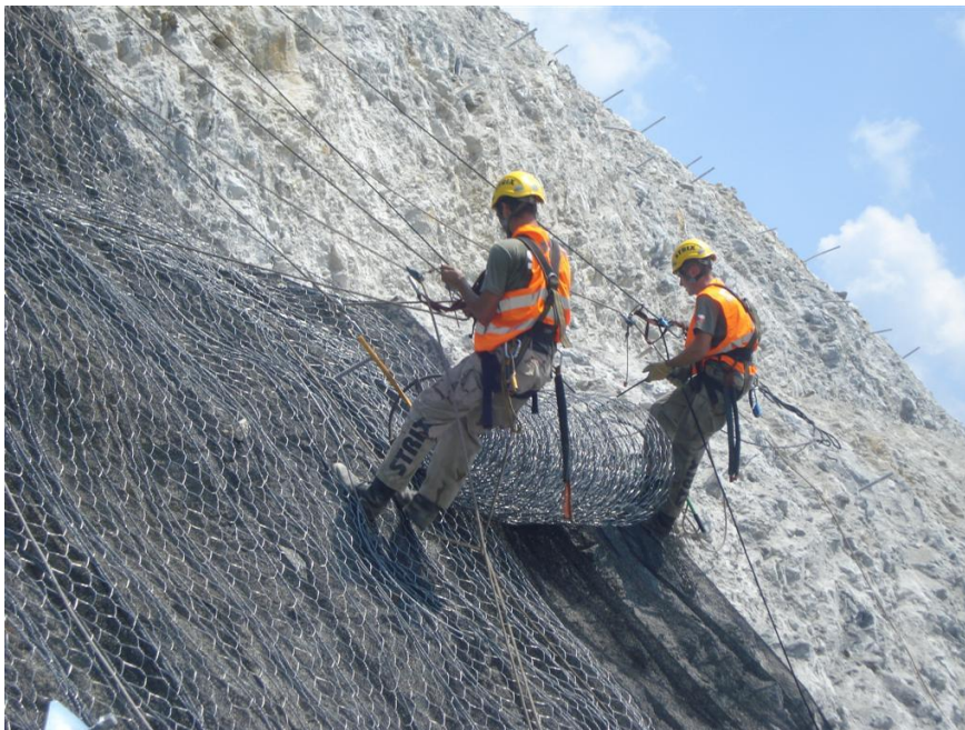
Figure 9 Installation of secured drapery Steelgrid HR30 kit (HR-Plate visible lower left) with mesh installed after the completion of anchoring operations
