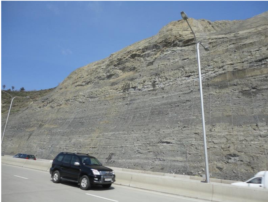
Figure 1 Rockfall protection offered to a road from a 90 m high unstable section of slope by Simple Drapery installation of Steelgrid HR mesh in Tbilisi, Georgia
