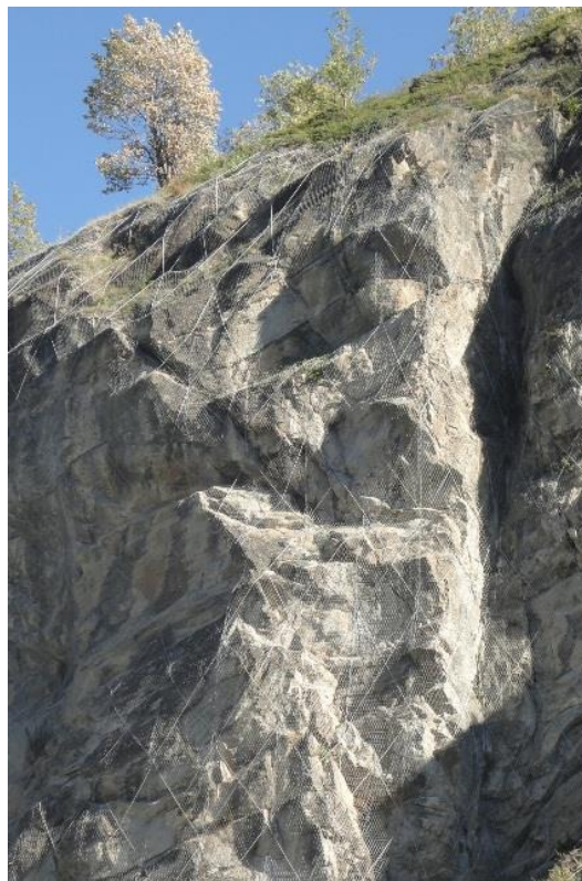
Figure 5 Secured drapery installation showing the mesh anchored back against the highly irregular topography of the slope face; Valle D'Aosta, Italy
