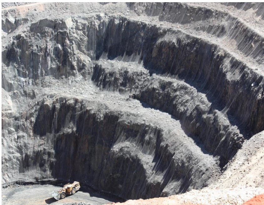
Figure 3 Simple drapery installation of Maccaferri double twist mesh, Rubicon Pit, Kalgoorlie
