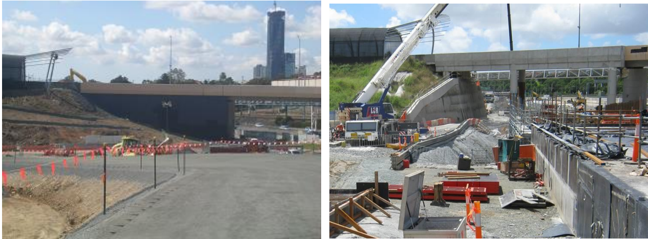
Figure 8 Anchored soil nail wall – before and after
