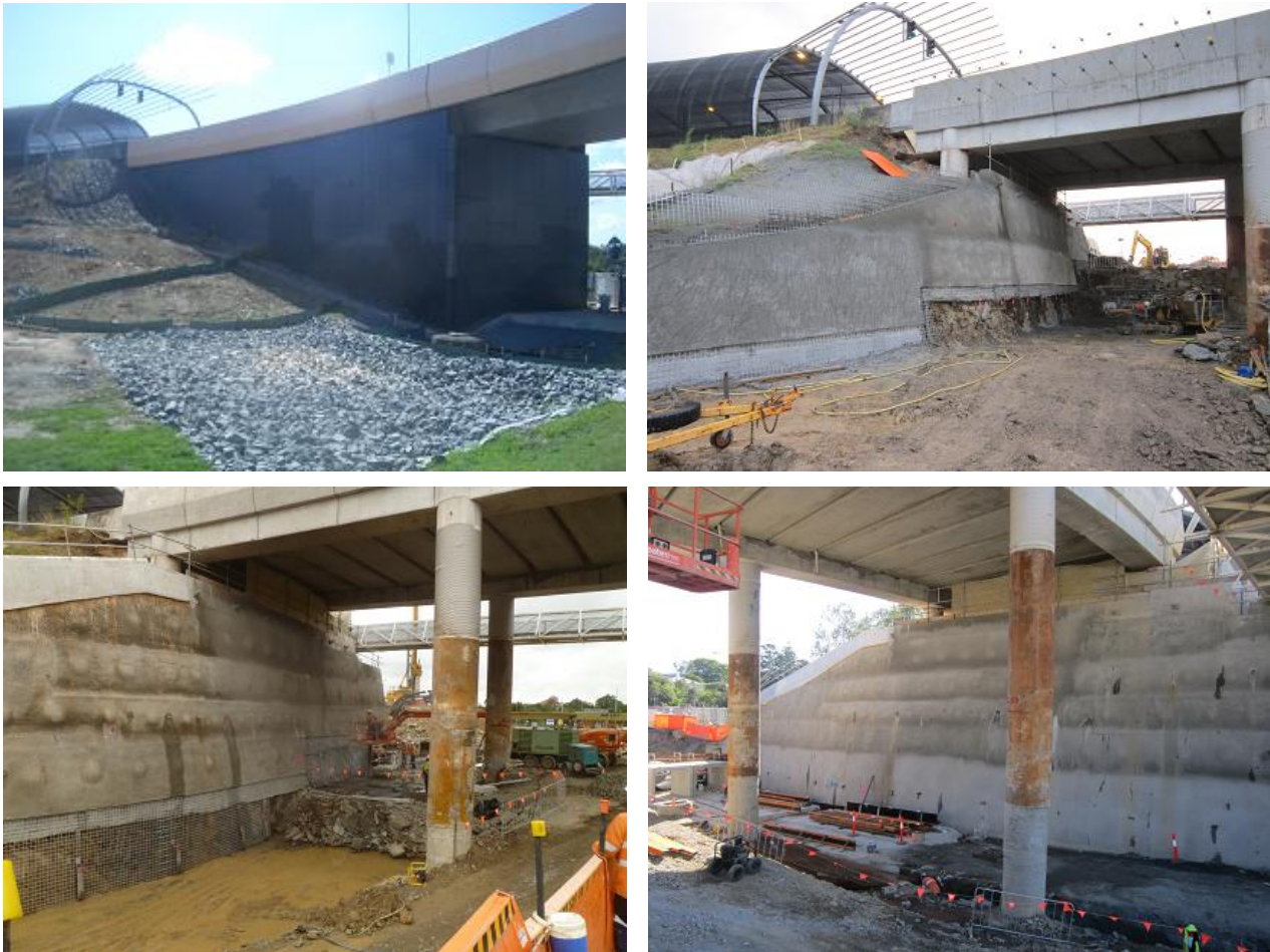
Figure 4 Soil nail wall during construction
