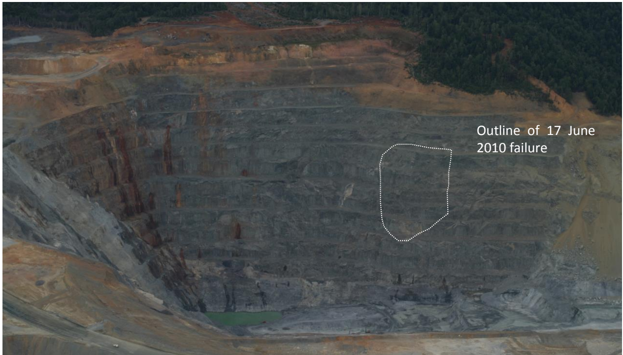
Figure 2 North Pit east wall
