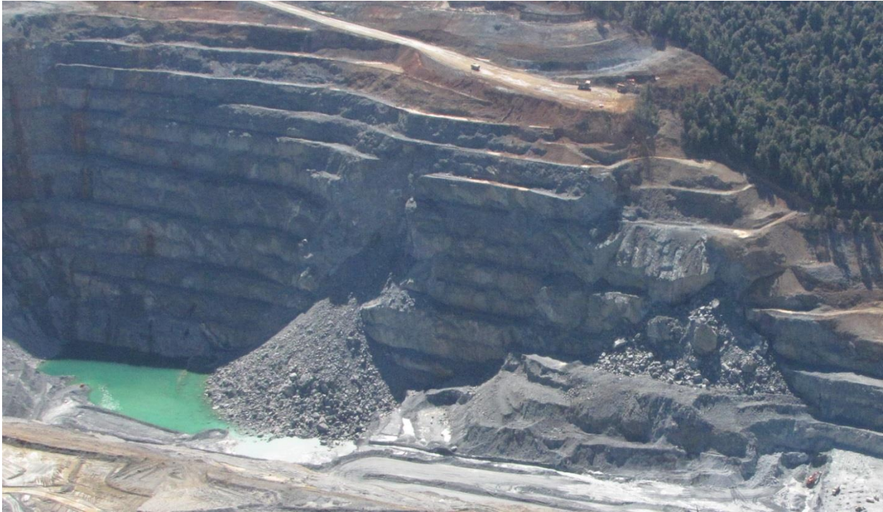
Figure 4 17 June (left) and 30 August 2010 failures
