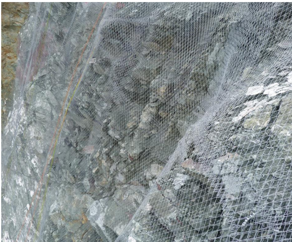
Figure 15 Highly fractured rock mass stabilised by TECCO®G80/4 mesh
