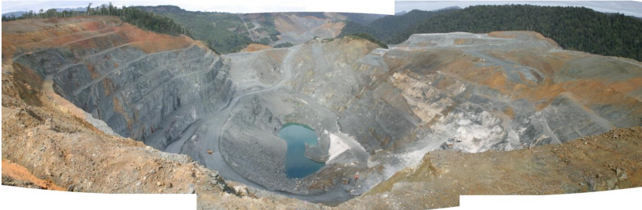
Figure 1 Photograph of North Pit (looking south)
