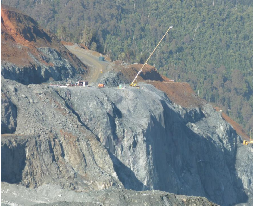
Figure 13 Mesh installation with 150 tonne crane
