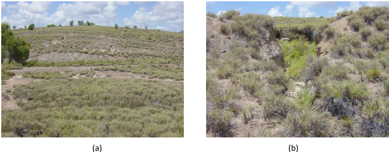
Figure 5 Images taken by Fletcher (2006) at Gregory coal mine three years after LFA transect data were collected at RehabG 1 ; (a) Illustrates how bank grading and steep slopes have led to the failure of the downhill slope; and (b) demonstrates pipe erosion caused by ponding in the constructed banks
