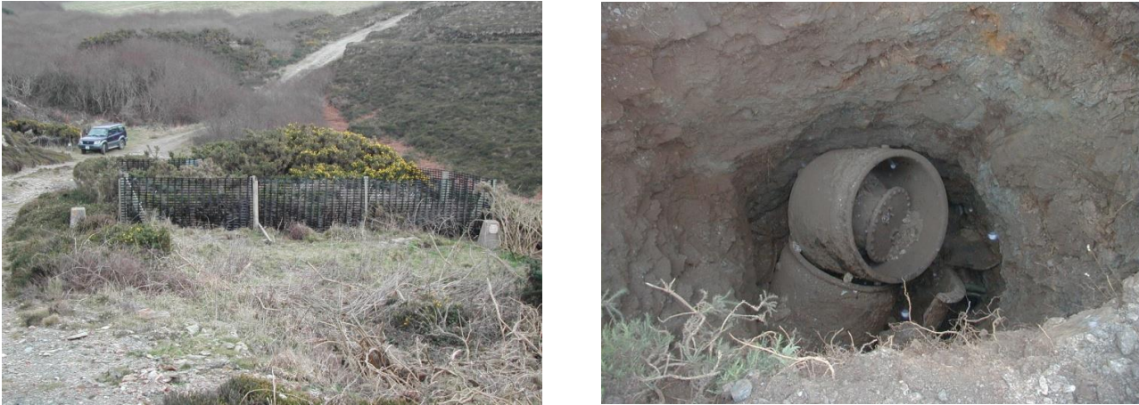
Figure 9 (a) Dump D (fenced area); and (b) excavation of the Ladderway Shaft
