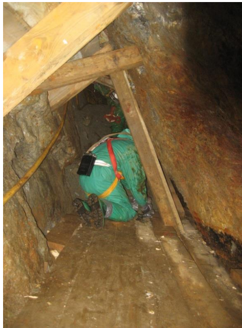
Figure 10 Stabilisation works above a winze
