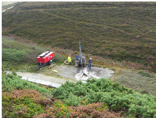
Figure 8 Looking from Dump D towards the drill rig
