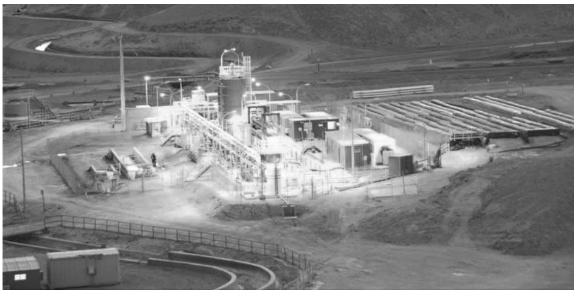
Figure 1 Overview of the pilot plant facility
